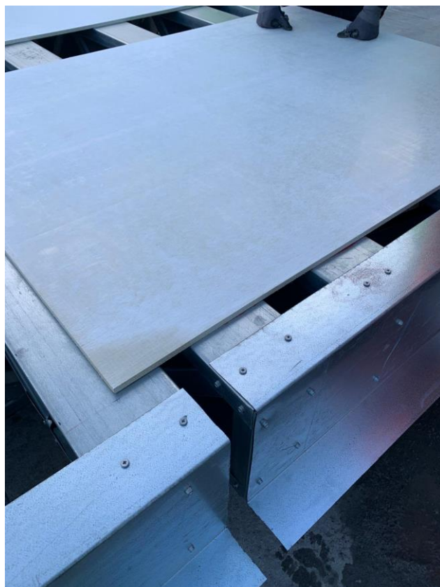
Photograph 2 – Sample during the construction – Ceiling Panels fitting in steel frame.
